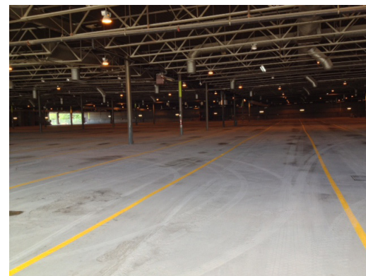
Victoria Park bus barn -post flood with newly painted lines
