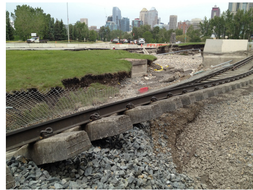
LRT tracks near Ertlon/Stampede Station
